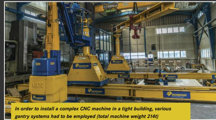
In order to install a complex CNC machine in a tight building, various gantry systems had to be employed (total machine weight 214t)
